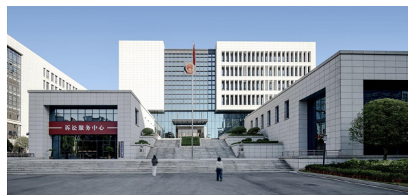
Figure 13: Main Entrance Plaza
