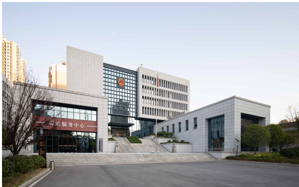
Figure 1: Huaihua Railway Transport Court
